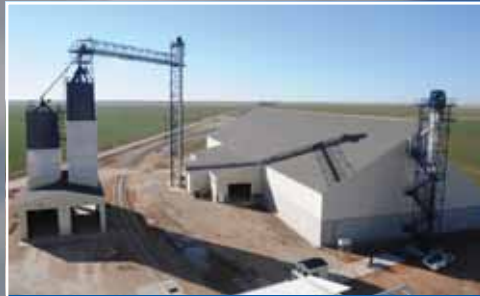
Incredibly efficient, high-volume railcar receiving.
