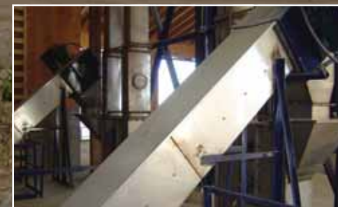
Totally-enclosed conveyor transfers conditioned material to leg.
