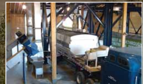
Multiple discharge lanes. Electric, telescoping dust spouts.
