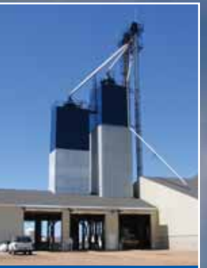
Holding tower & blend tower each have separate lanes.
