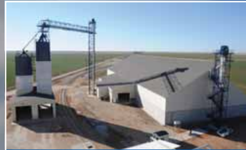
Incredibly efficient, high-volume railcar receiving.
