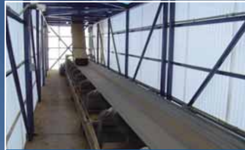
Totally-enclosed truss protects material from the elements.
