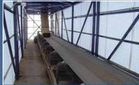
Totally-enclosed truss protects material from the elements.
